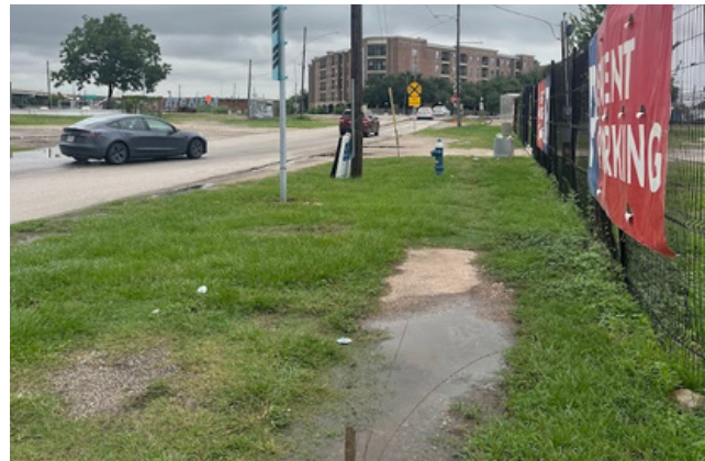
Many sidewalks in the project area are unpassable, such as this one on Hutchins Street in East Downtown
